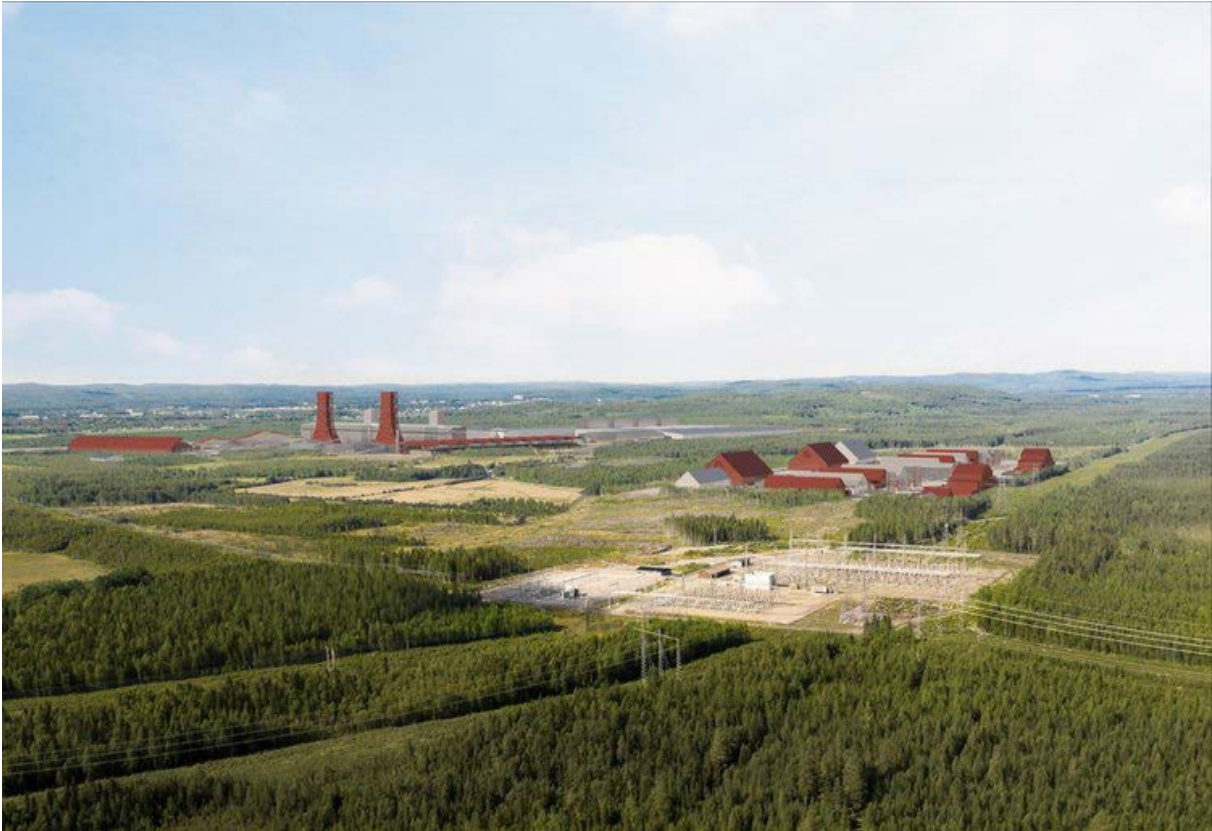
H2 Green Steel, preview of Bodø facilities.
