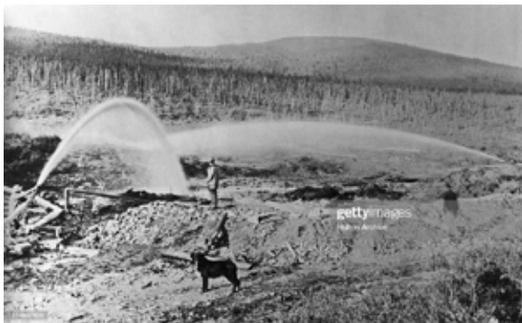
Photo 32. A hydraulicking operation to mine a placer deposit. From Getty images, Hulton Archive.
