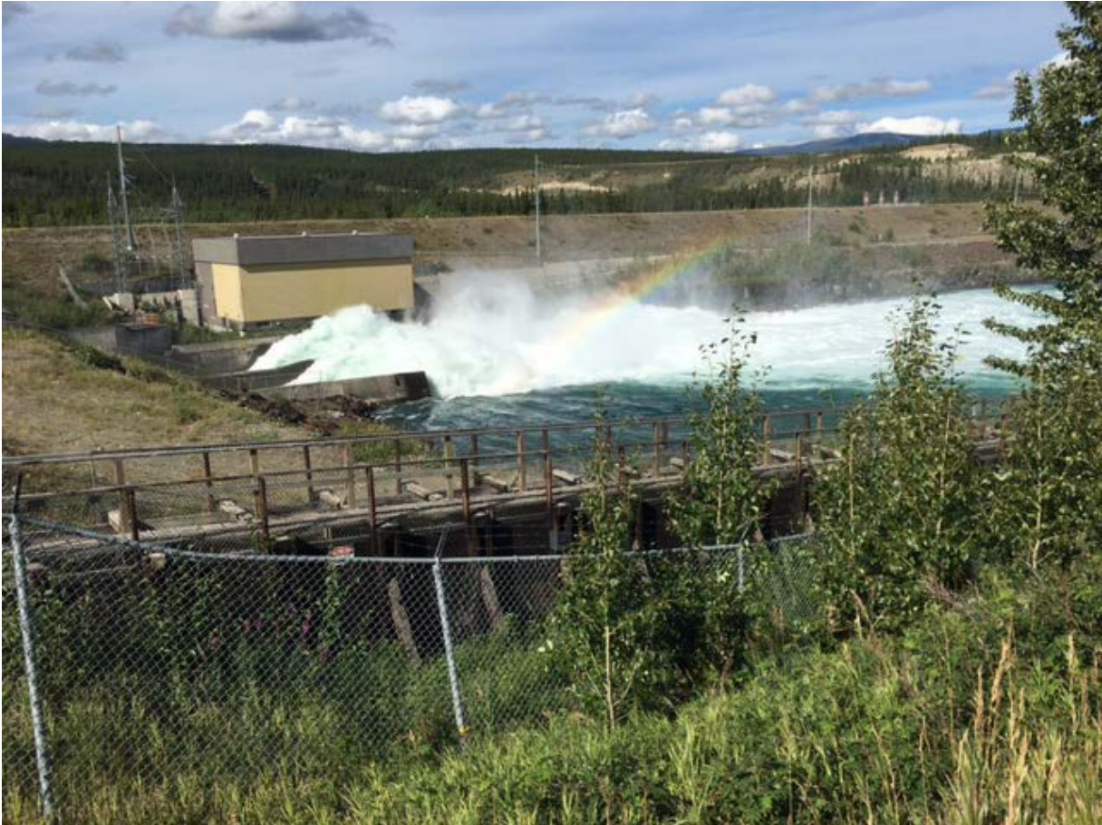
Photo 4. The present-day dam, spillway, turbine #4 and the fish ladder at the Whitehorse Power Plant. Photo by the author.
