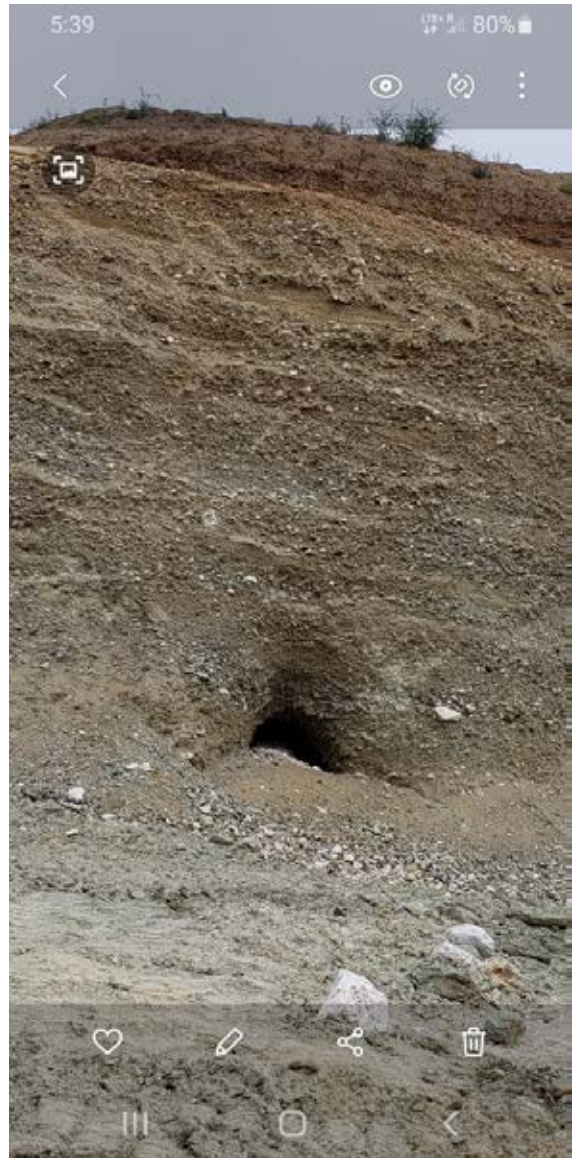
Photo 31. An old timer's tunnel exposed at the Chechako Hill Mine. Photo by the author.
