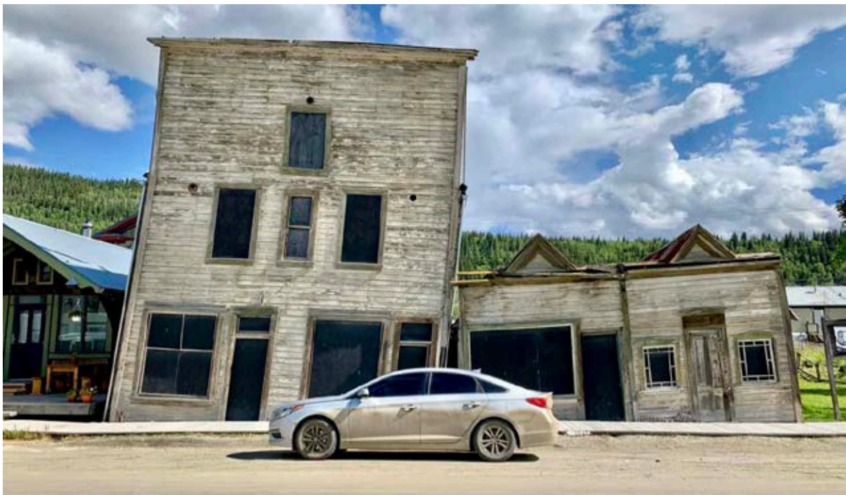
Photo 18. Melting permafrost makes some buildings in Dawson City uninhabitable for safety reason. Photo unknown.
