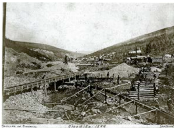
Photo 26. Mining by hand and sluicing in 1899 in the rich Eldorado Creek in the Klondike. In the back ground the small village where the miners lived. Photo Sam Dunn.
